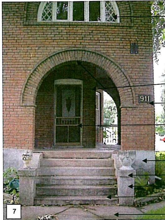
Front Entry and Stairs
