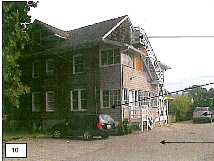
South elevation of building.
