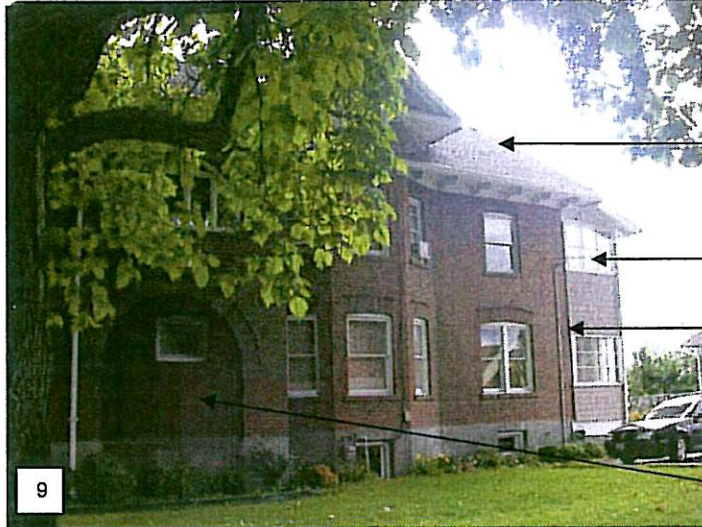
West elevation of building.
